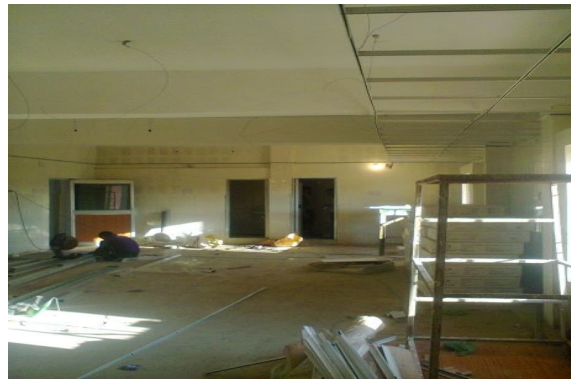
Construction of NCD Complex, Koraput as on 01.12.13
