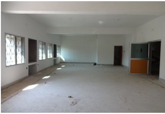
Construction of NCD Complex, Bolangir as on 01.12.13
