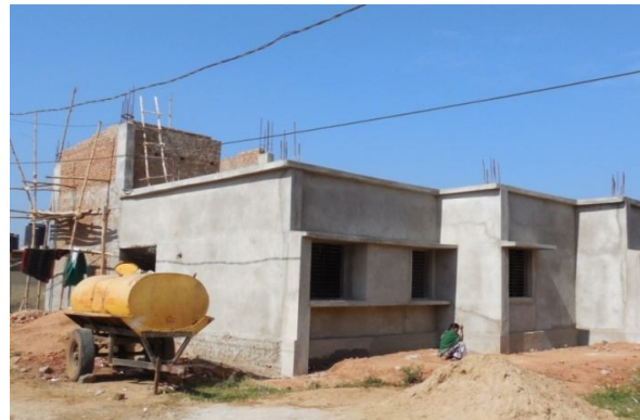
Construction of NCD Complex, Nabarangpur as on 01.12.13
